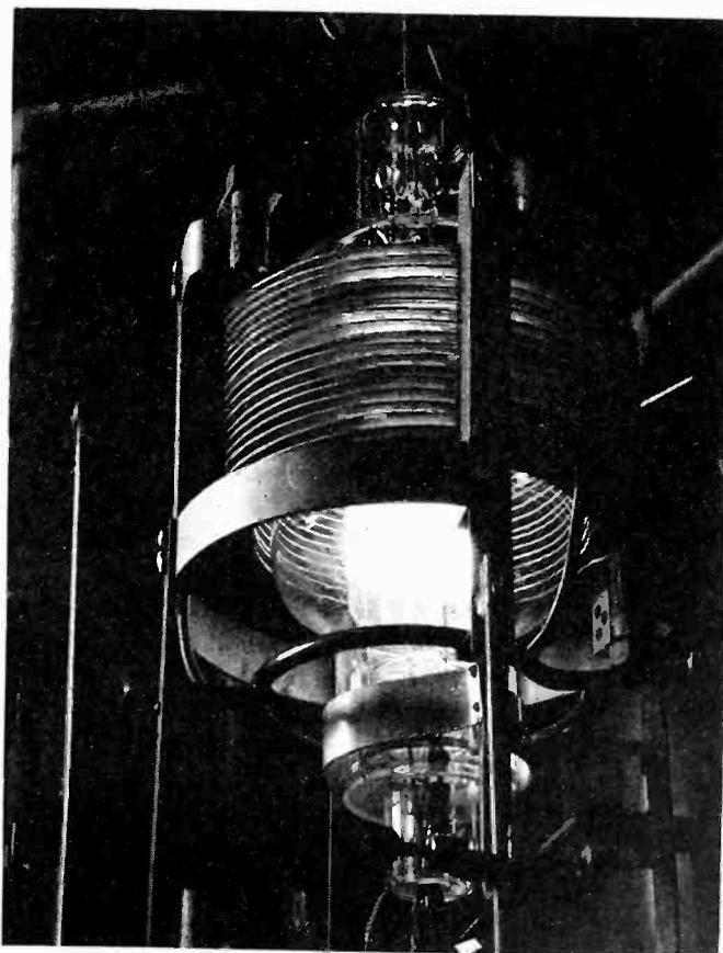
**Bombarding a power tube—an important process—in the Bell Telephone laboratories.**
